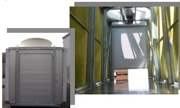
\*As an option; a hydraulic lifting table allows removal of the motor/fan set in complete safety, without means of other lifting equipment. Also, easy handling of the humidifying pads is possible, without any lifting/ handling tools.
